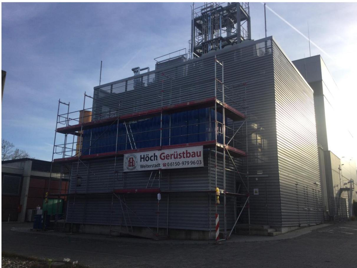
**Figure 13: Image of the novel gas treatment plant (background) and the two RWE test rigs (lower container behind cladding: fuel synthesis test rig, upper container: gas treatment test rig).**
