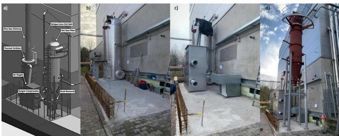
**Figure 12: Concept (a) and progress at the construction site (b-d) of the novel syngas removal unit at the 1 MW<sub>th</sub> pilot plant facilities in Darmstadt.**
