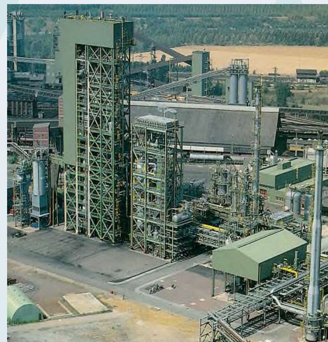
HTW Demonstration Plant Berrenrath (1986-1997)
