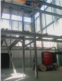
Erection Pilot Plant
