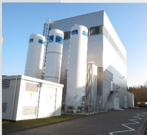
Commissioning Pilot Plant
