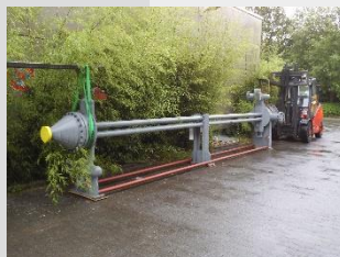
Erection HTW™ Gasifier
