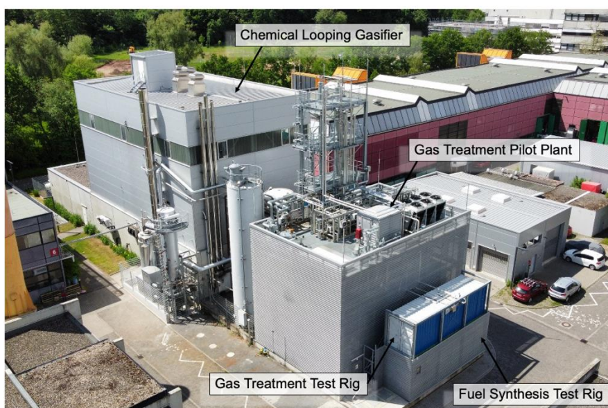
Figure 4: Overview over the 1 MW th pilot plant at TUDA, consisting of the Chemical Looping Gasifier, Gas Treatment Pilot Plant, Gas Treatment Test Rig, and Fuel Synthesis Test Rig.
